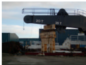
If you see an unsafe act or condition within the harbour report it!
