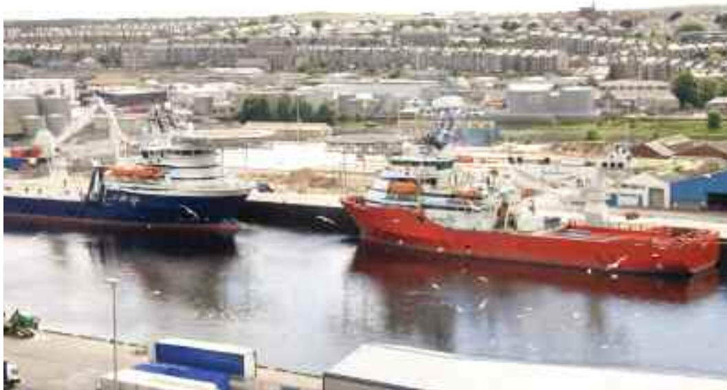
The upgraded Albert Quay West and, beyond, Point Law Peninsula where a new yard was completed in 2007.
